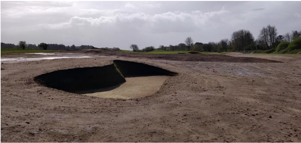
Figure 2 Reprofiled Fairway during construction
