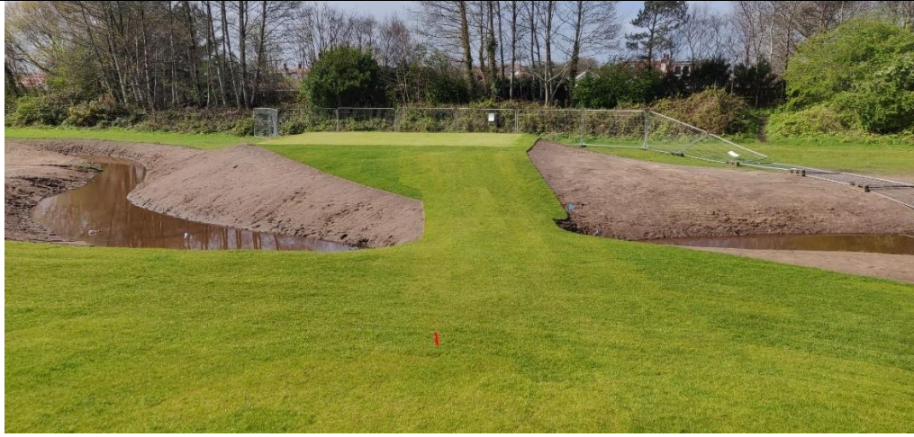
Figure 3 New 2nd Green and Drainage Ditches
